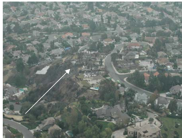
Arrow pointing to the same slope after the Freeway Complex Fire showing the tragic loss of homes along the ridge
