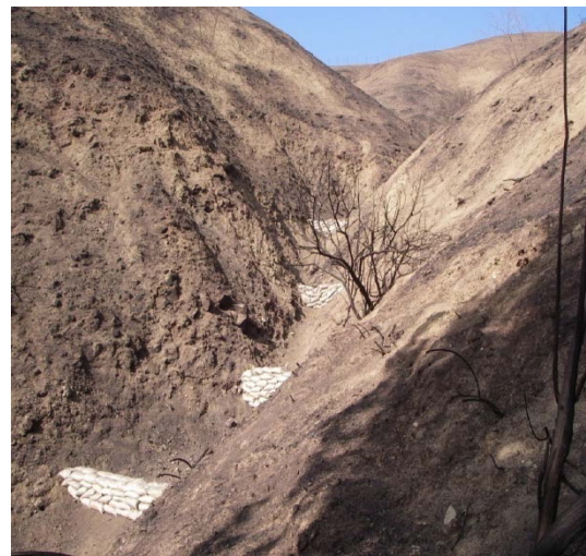
Sand bags in place west of Banyon Rim.
